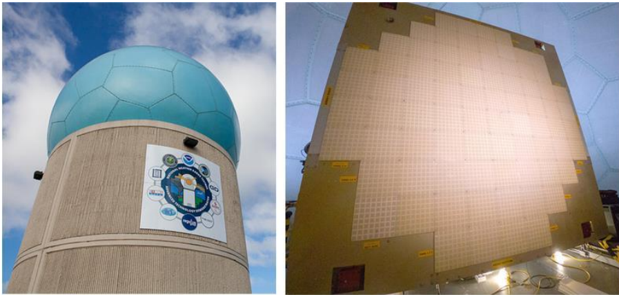
Fig. 6.2.1. ATD site and the antenna under the radome.
