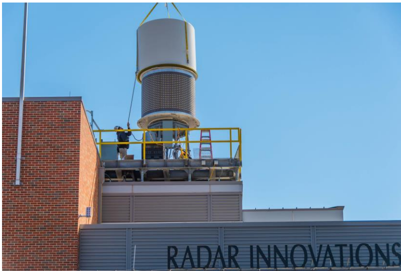
Figure 7.2: A picture of CPPAR being installed on the top of RIL
